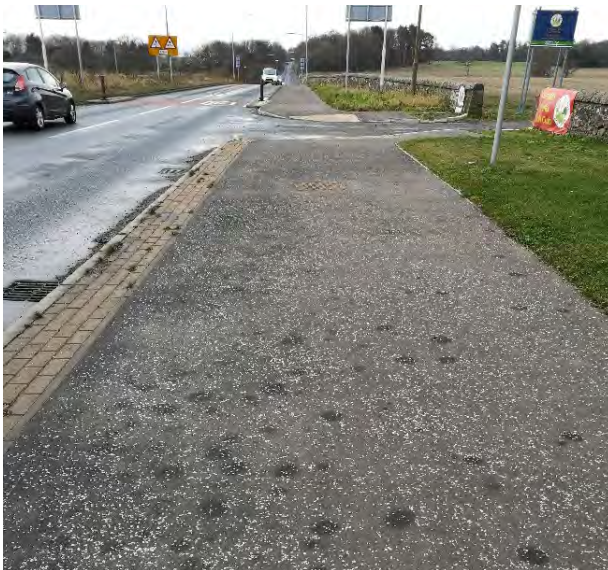
Figure 13 – Traffic calming build-out on B8000
